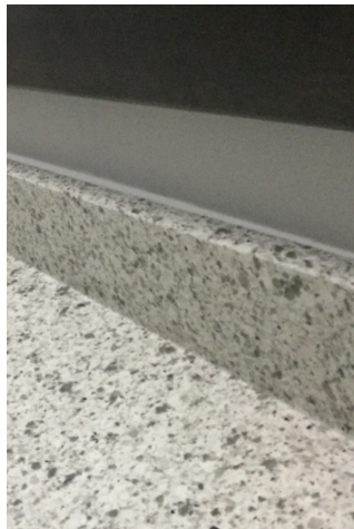
Bow corrected with caulk
