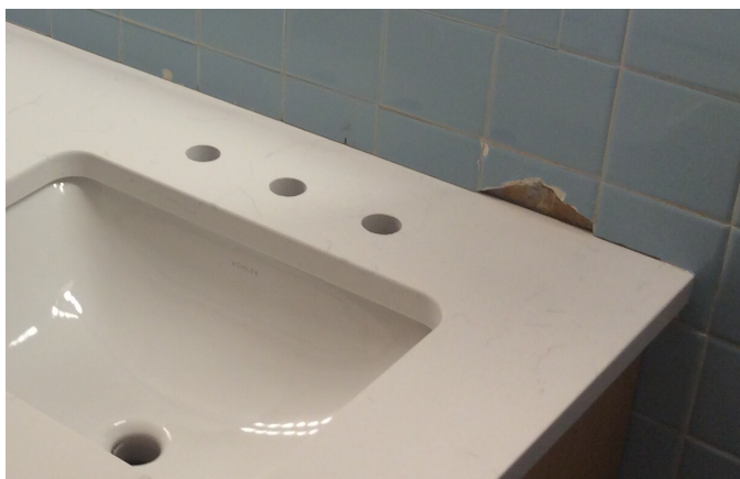
Damage to existing tile
