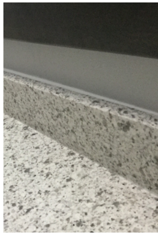
Bow corrected with caulk
