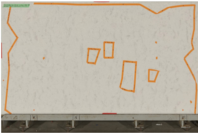
UNEVEN TEXTURE The orange tape indicates the texture - some areas have a high concentration of texture, while others do not.
